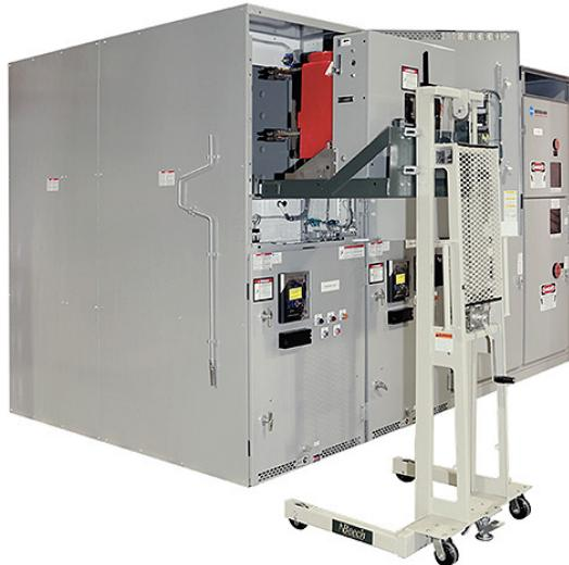
*To ensure the safety of personnel servicing the equipment, all Benshaw medium voltage switchgear offerings include a rack-out circuit breaker design. A remote breaker control panel and arc flash sensing options are also available to further enhance personnel safety. In addition, Benshaw offers a full metal-clad switchgear solution.*
